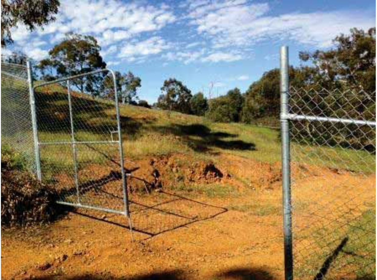
Plate 5: Missing gate at a revegetation site
